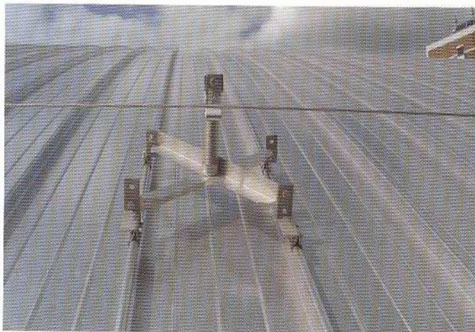
Intermediate Bracket for Aluminium Seamless Roof
